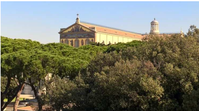
View of St Paul-Outside-the-Walls from the Beda College
